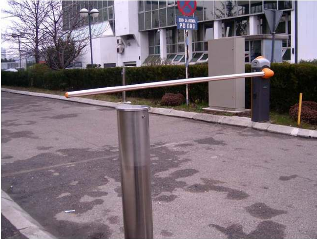
Barrier controlled by the Proximity terminal with two readers on the stainless steel pillar
